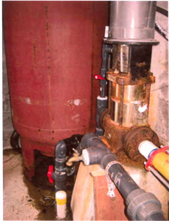
FIGURE 3.6.3.2 Deady Street Pump Station
